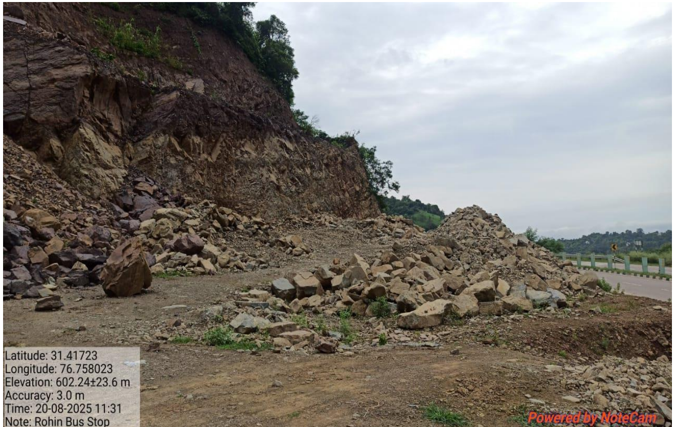
Photographs No. 01 : Shows the Status of Excavation Site No. 1.
