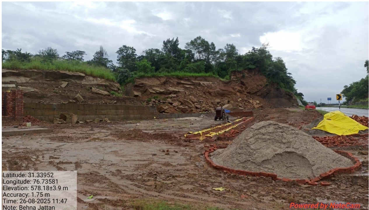
Photographs No. 01 : Shows The Status Of Excavation Site No. 2.
